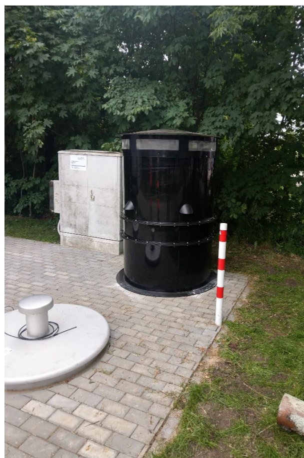
Figure 8: OCU in Germany with Iron Hydroxide 1 st stage and activated carbon to remove VOCs 2 nd stage, flow 370 m 3 /h, H 2 S 350 ppm, humidity 90 – 100 %
